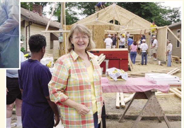
Area Lutheran Habitat for Humanity build
